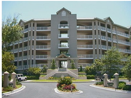
Hampton Entry / Building
