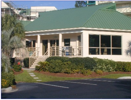
Villamare Fitness Center
